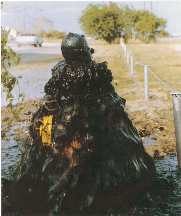
1. Poly Pig exits potable water piping system after traveling 1,300'.
